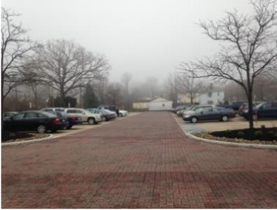
We then visited the South Euclid City Hall where the city converted its parking lots to include permeable pavers to increase groundwater filtration. The front lot is totally permeable; in the lot, only parts were retrofitted. The aim is to keep the surface as flat as possible so the water drains down through the 30-inch stone base installed below it. Dirt collects over time and it needs to be swept out or vacuumed to keep out mud.
